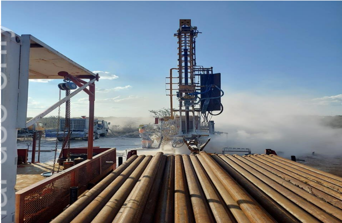
Figure 1. Drilling at Serowe-3.5B (Source: Botala)
