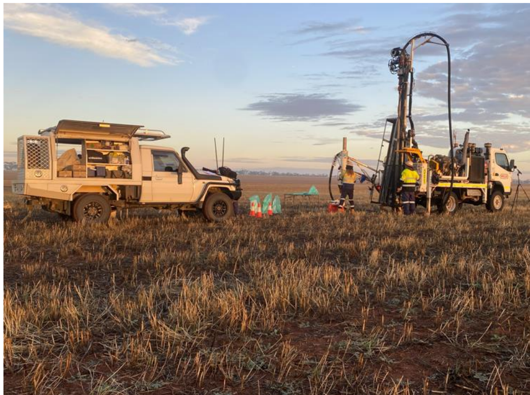
Photos from the drilling activity which commenced during the quarter
