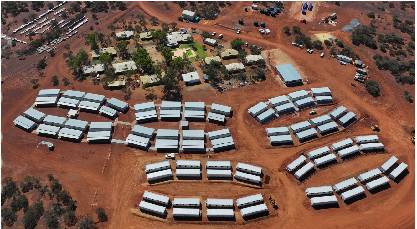
Figure 4 – Camp expansion preparation works advancing
