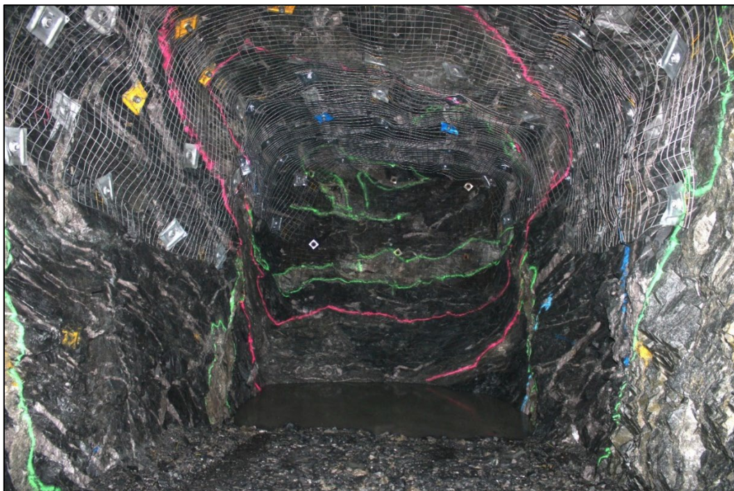
Photo 2 – 2341mRL level access (cross section view)
