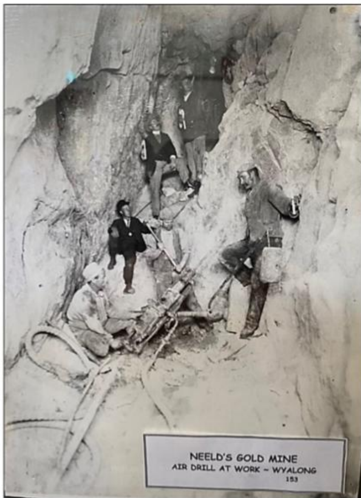
Figure 3 – Historical mining within a ~3 metre stope at Neeld’s Gold Mine 6
