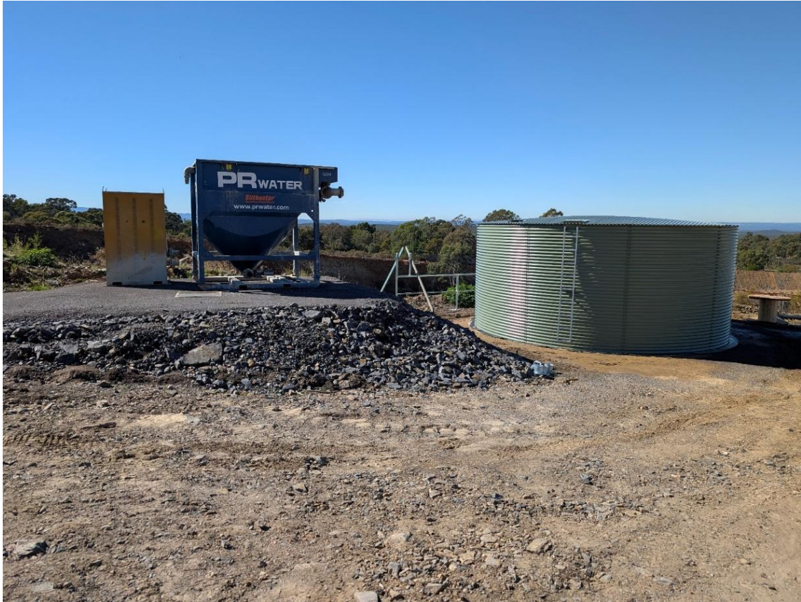
Figure 2. Water tank and clarifier installed in position
