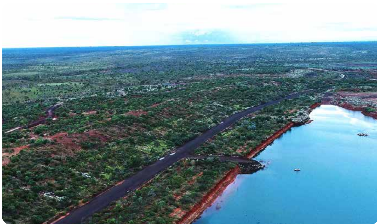
Figure 4: GoGo and Xhosa WRDs (looking South East)
