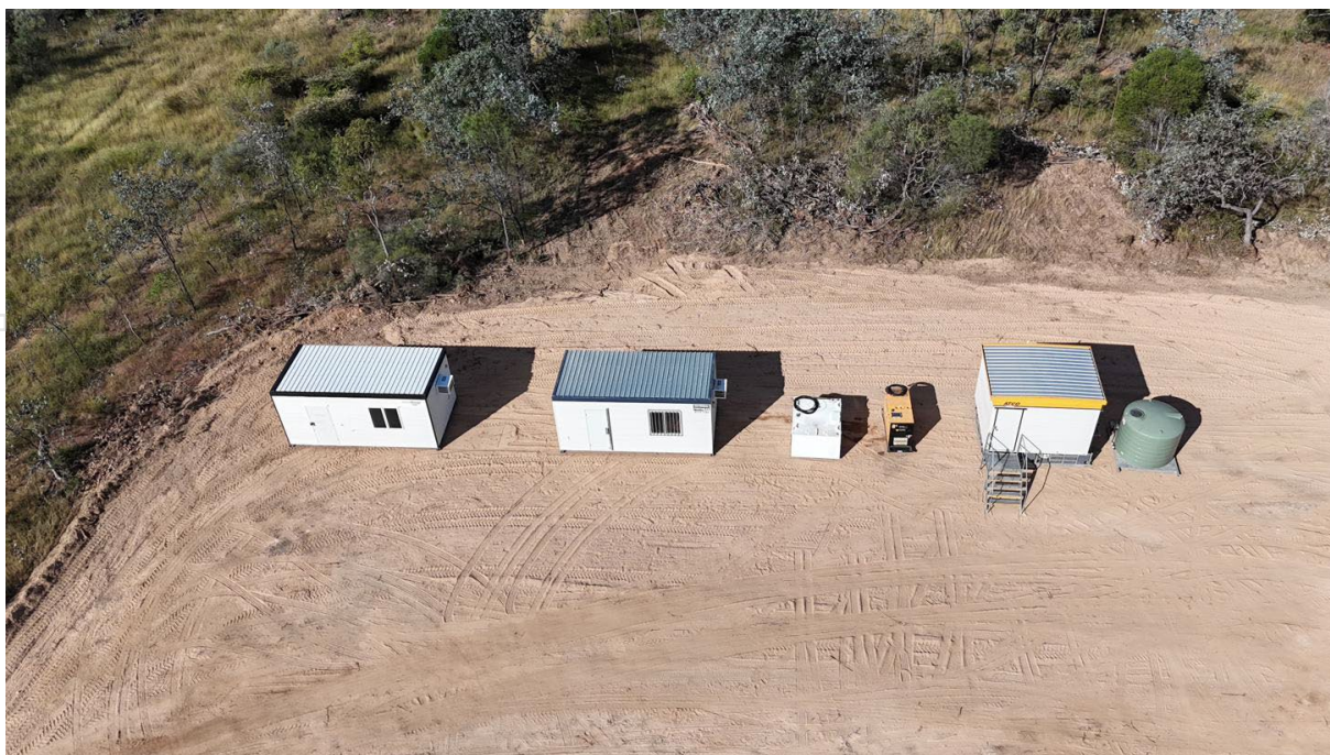
Figure 3: Podosky site establishment – site offices, generator and water infrastructure in place (22 April 2026)
