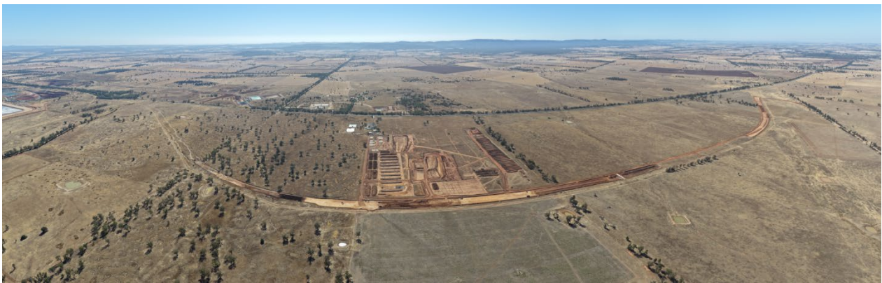
Newell Highway works looking east.
