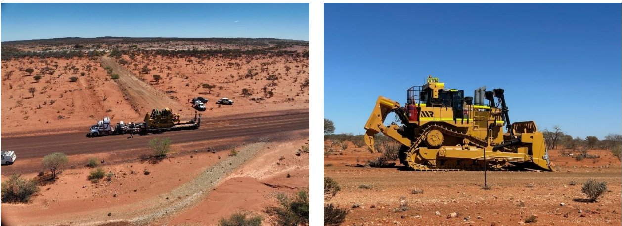
Figure 2 - Mobilisation to site and site preparation activities
