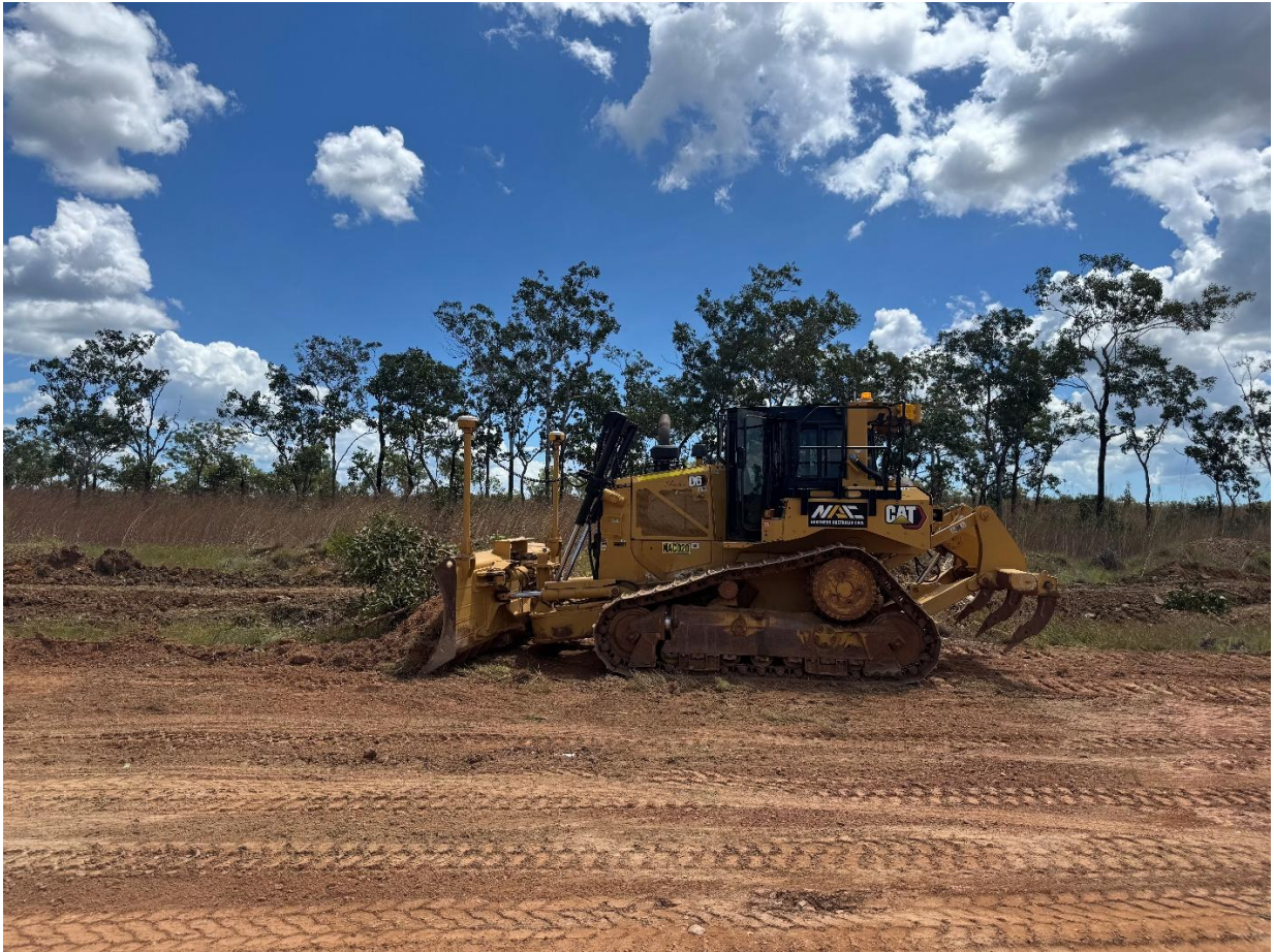
Figure 1 BP33 early works underway
