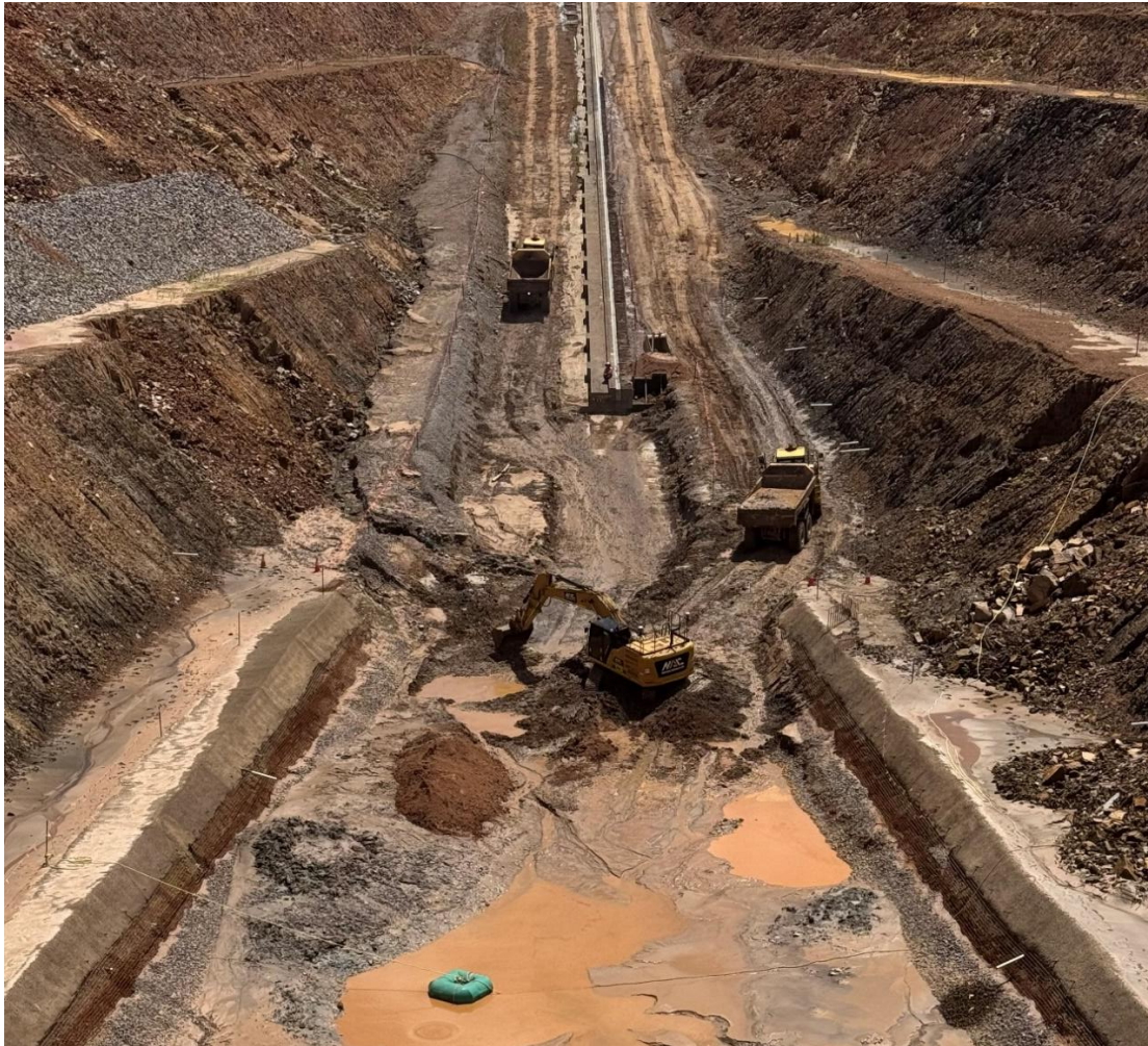
Figure 2 BP33 boxcut and infrastructure site works post Quarter end
