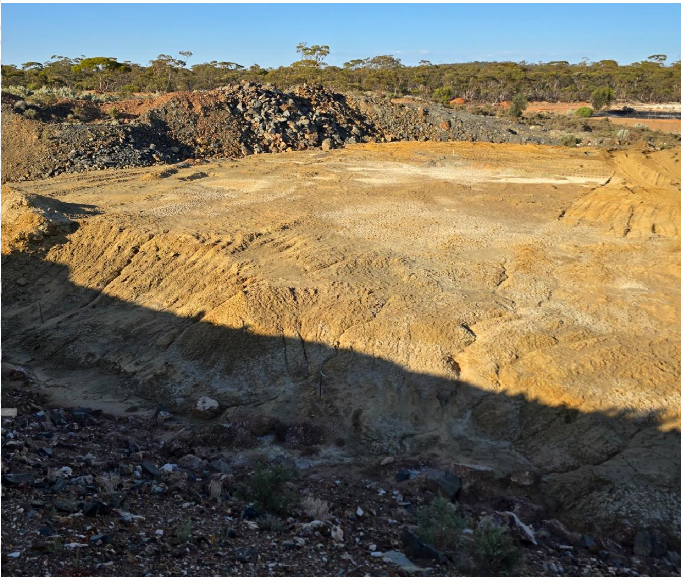
Figure 3: SW Tailings Dam
