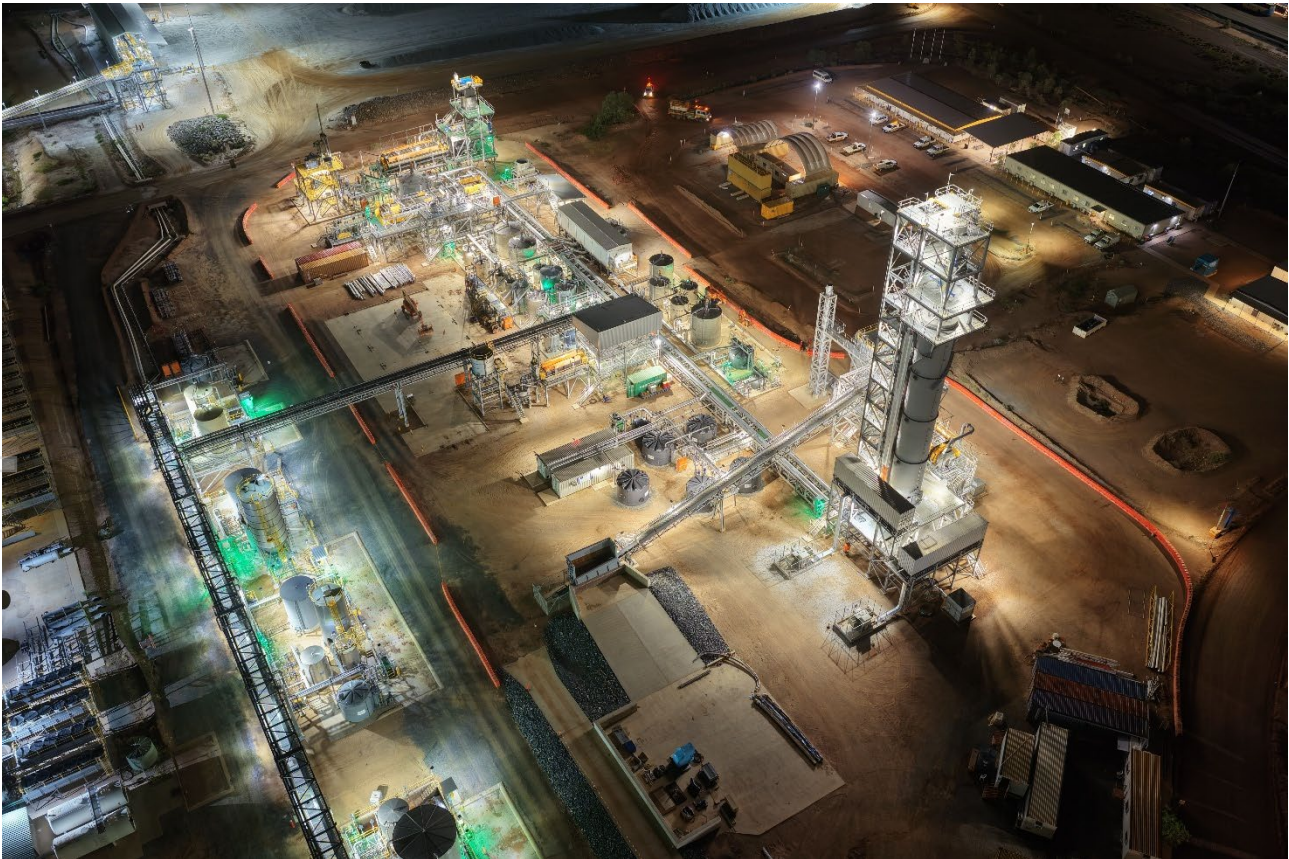
Image: Mid-Stream Demonstration Plant as at 2 April 2026.
