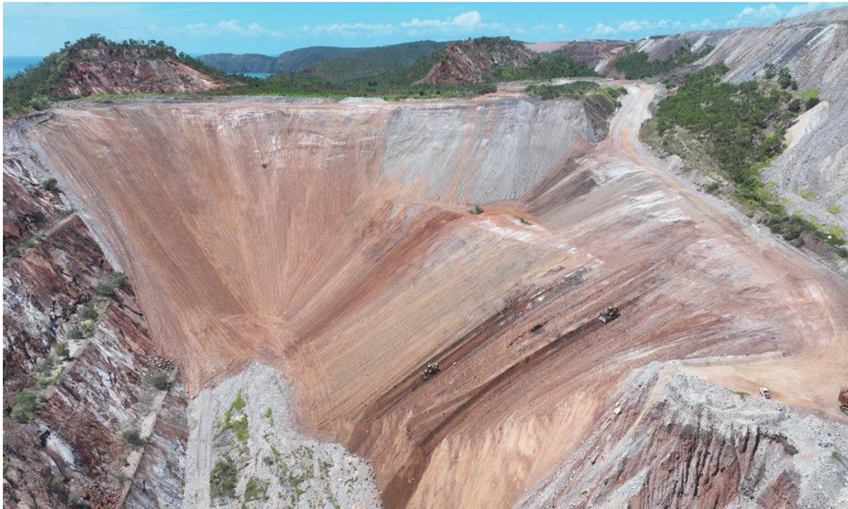
Figure 2 - Rehabilitation earthworks at Mullet Pit on Koolan Island, April 2026.
