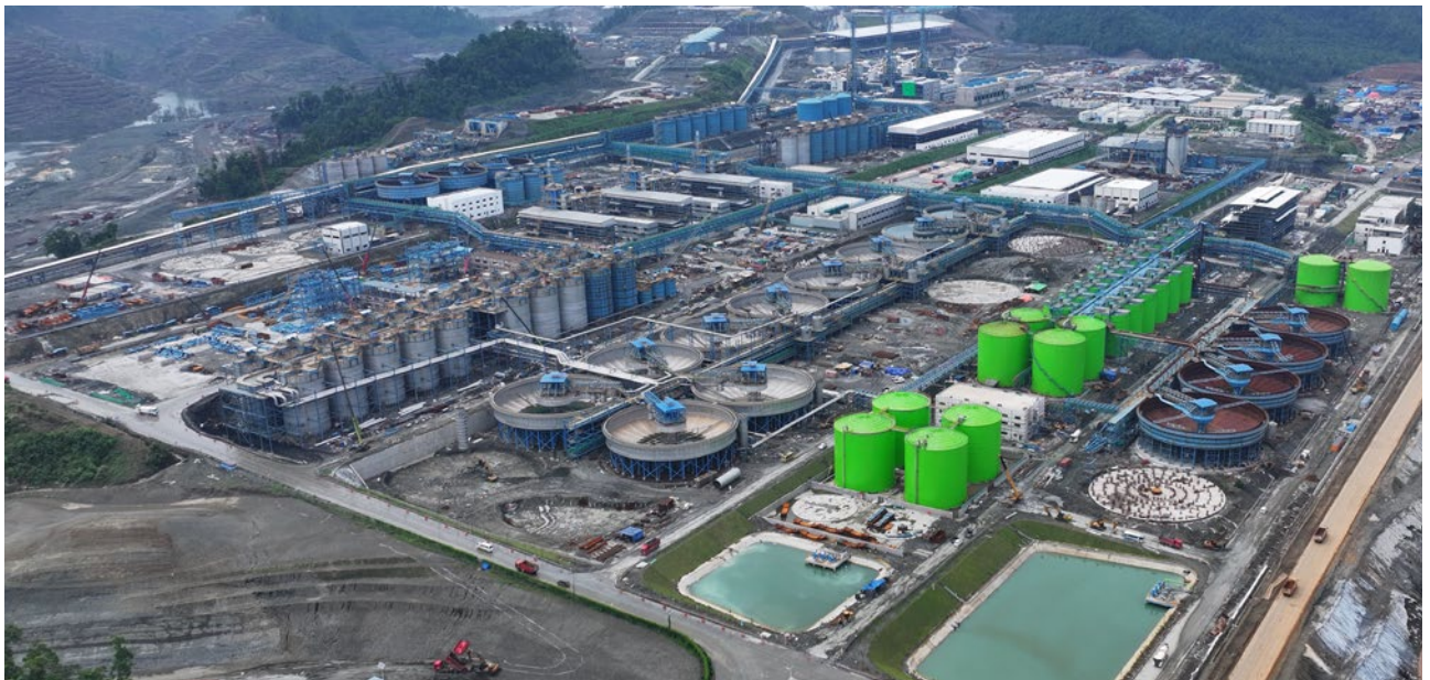
ENC HPAL smelter construction progress
