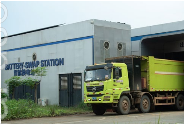
EV battery swap station and electric loader
