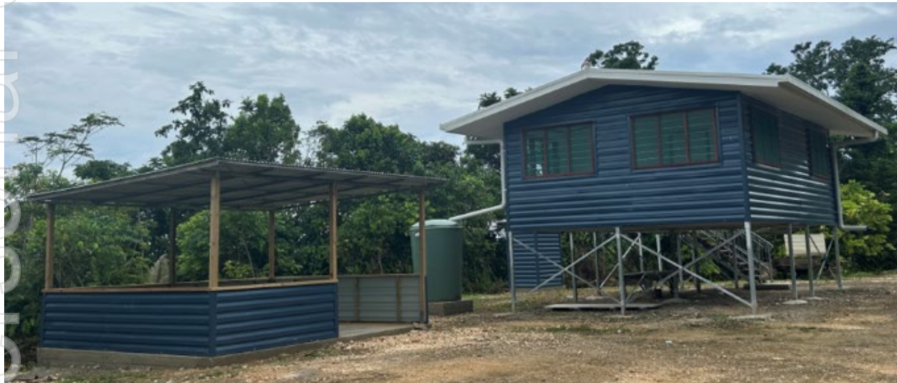
Relocation house completed during the reporting period
