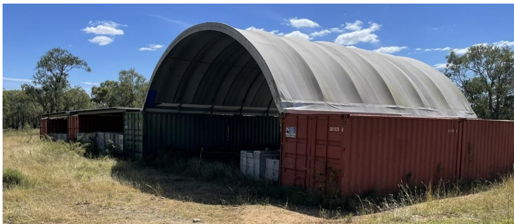
Figure 7 Monto Project, Field Camp and Core Storage Facility, April 2026
