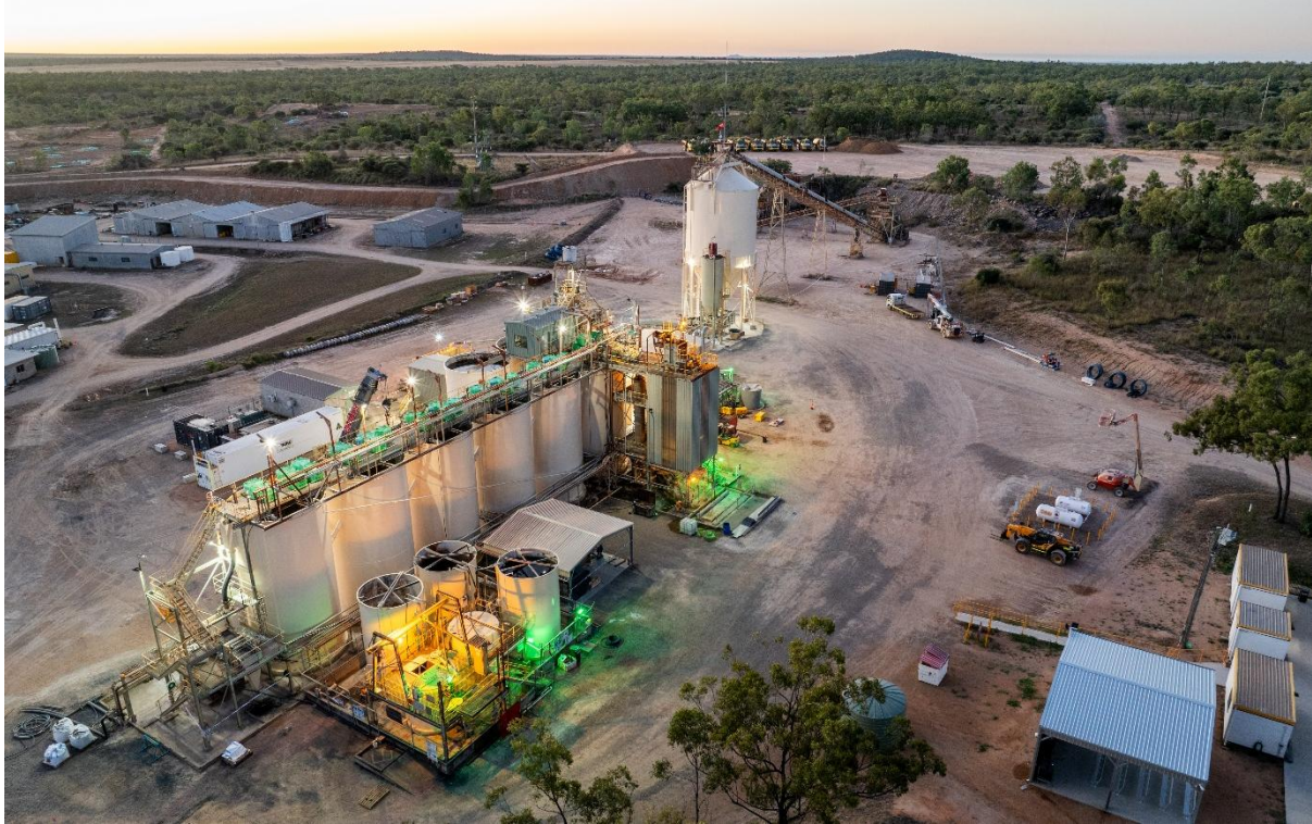
Figure 2: Overview of Blackjack Plant
