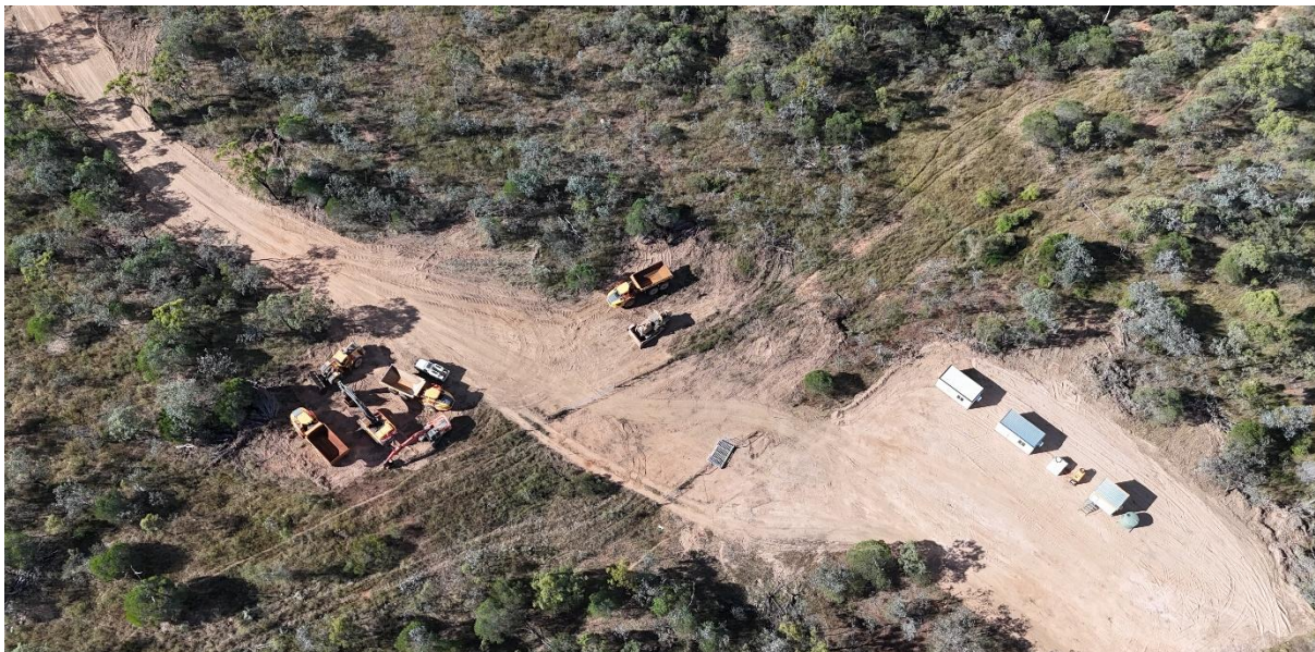
Figure 7: Podosky Site Buildings and Mining Fleet Mobilised (post quarter-end)
