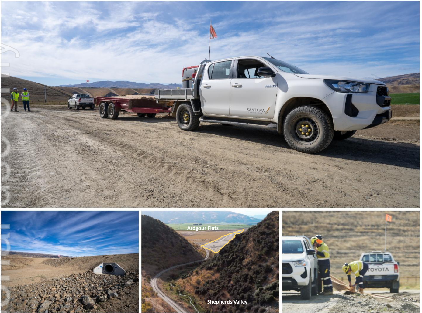
Figure 3. Santana construction teams executing permitted early works at the mine entrance on Ardgour Flats
