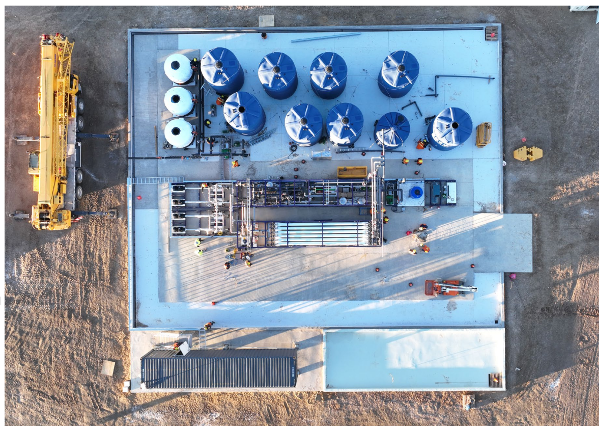
Figure 2. HMW site team working on the installation of the filtration plant.
