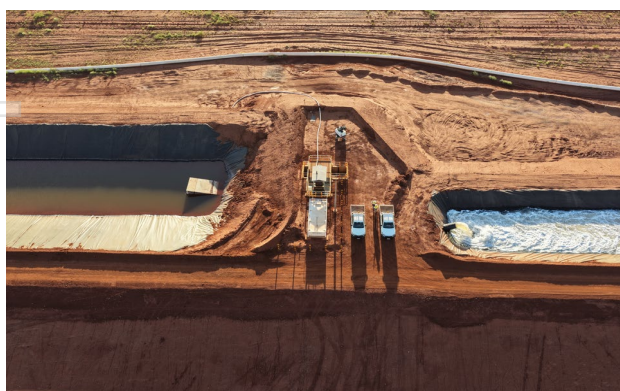
Figure 5: Lift station two commissioning
