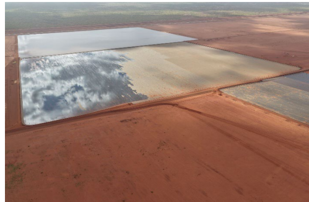
Figure 3: Filling of the second crystalliser
