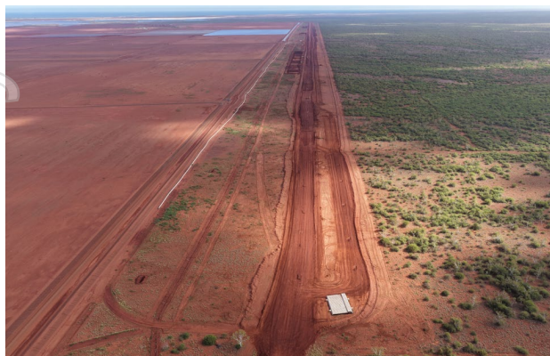
Figure 7: Pilbara Ports road
