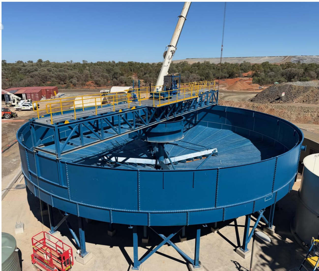
Photo: Tailings Thickener installation at Peak (March 2026)
