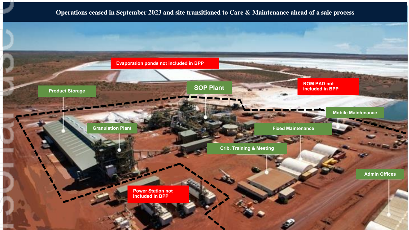
Figure 13 – Photograph of the Beyondie Potash Project in 2023 when in operation by Kalium. The assets include a fully constructed processing plant, site offices and maintenance infrastructure. Specific plant components include, KTMS crushing circuit, Kainite conversion circuit, column flotation circuit, liquor cooling heat exchangers, evaporative cooling circuit, product separation centrifuges, SOP recovery and granulation units, RO water plant and a bulk storage shed. 1
