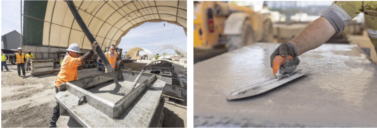
Figure 3 & 4: Wind farm concrete trials - 50% AusPozz™ mix design
