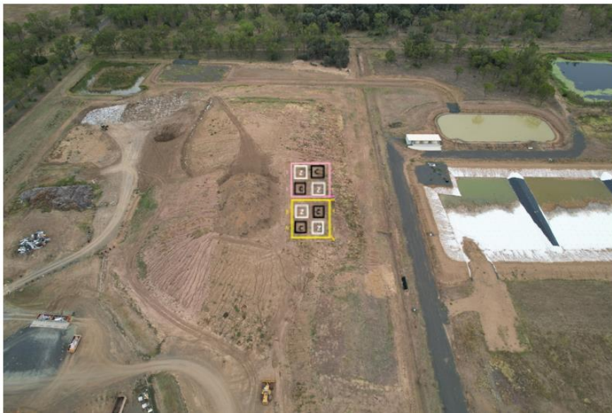
Figure 5: Zeotech's Methane Control Program at a NBRC Landfill
