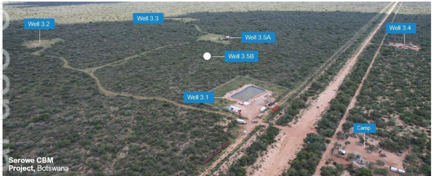
Figure 3. Project Pitse showing commercial well pilot locations.
