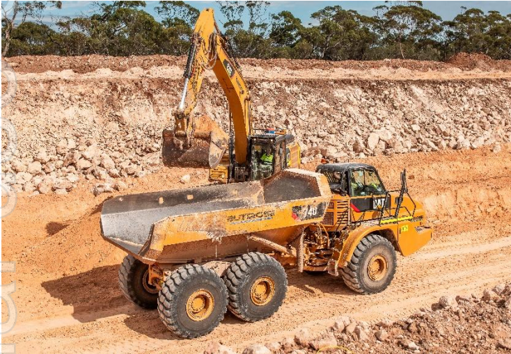
Excavation of the stormwater pond
