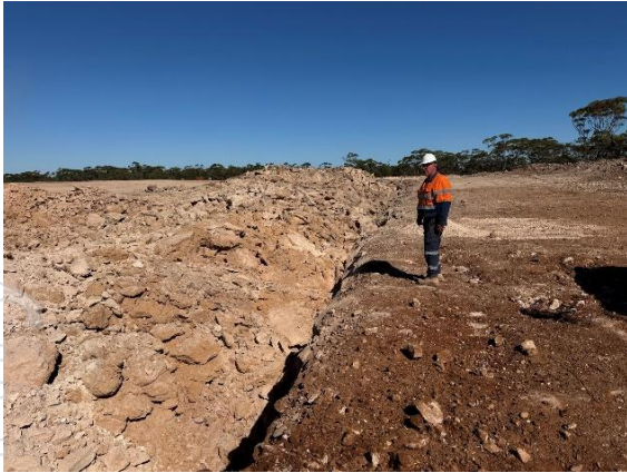
Post-blast inspection of the stormwater pond
