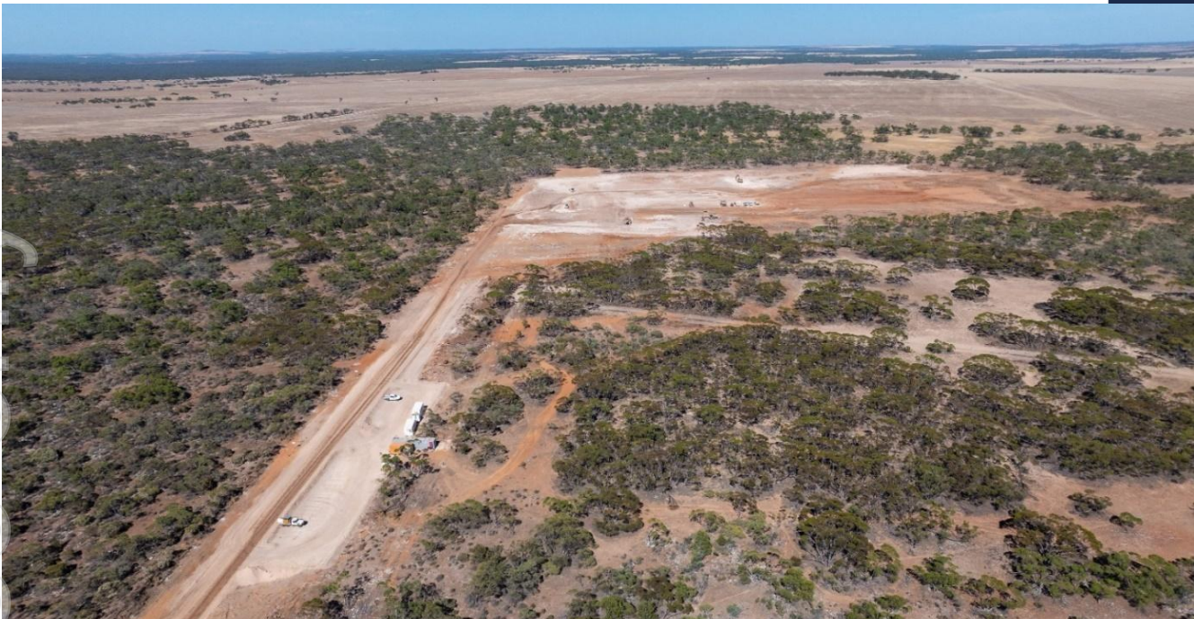
GWP mine access track leading to Stage 1A+ Processing Plant Pad
