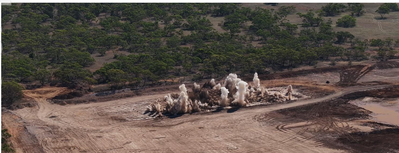
Controlled blasting of the stormwater pond in progress
