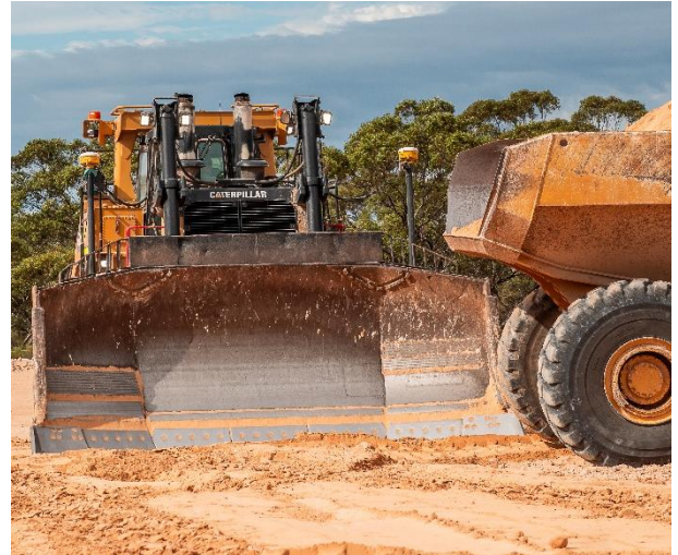
Finalising the processing plant clearance
