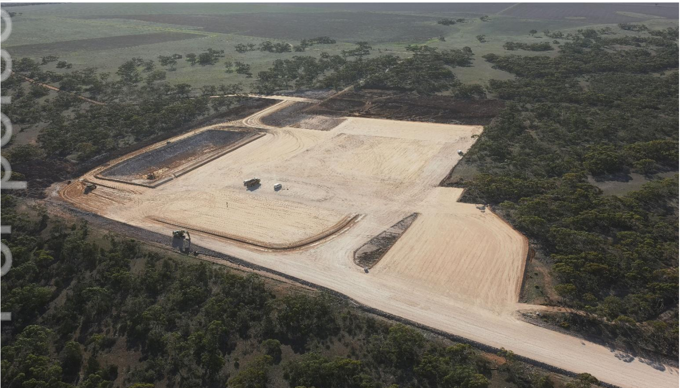
Processing Plant Pad Early Works Construction Completed
