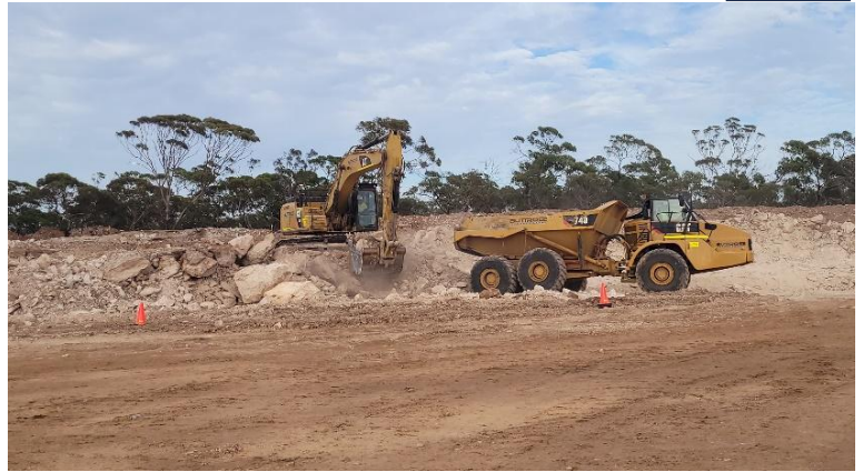
Excavation of stormwater pond following blast
