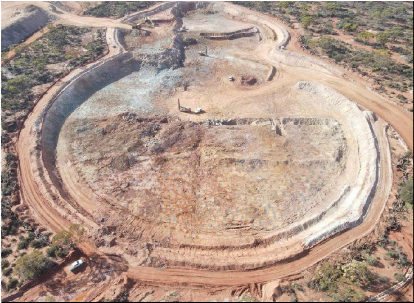
Figure 4: End of March 2026 - mining the Lady Herial Pit 315-310mRL & commenced drilling & blasting 305 RL bench.
