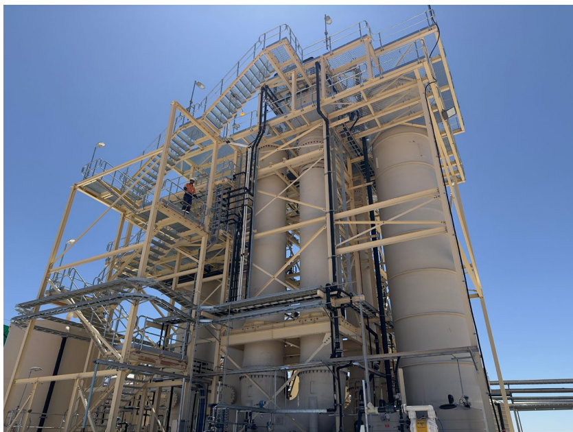
Practical completion of the CLEAN-IX® U-Column system reached.
