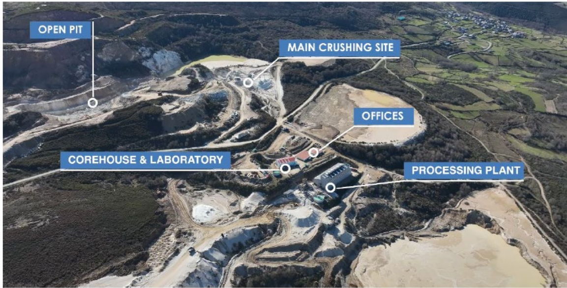
Figure 1: Overview of existing infrastructure at the Penouta mine
