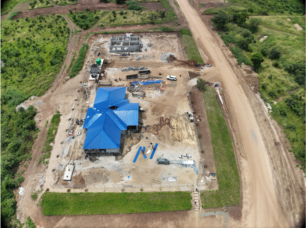
Picture 4. Aerial view of the site administration precinct under construction including the admin building and site medical clinic
