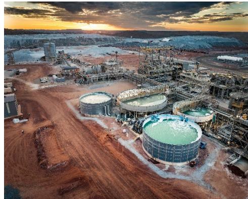
Figure 4: Aerial view of process plant
