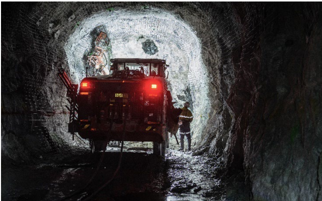
Figure 1: Jumbo advancing development of the underground mine
