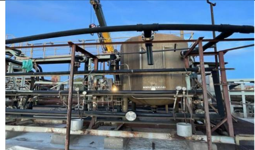
Installation of Spintek filter tank
