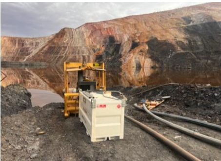
Pit dewatering pump
