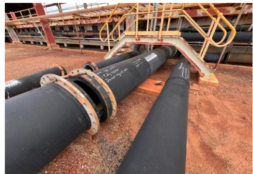
Reinstallation of piping to EW
