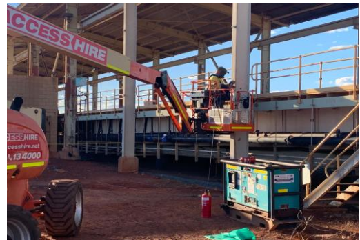
Refurbishment of gantry crane supports
