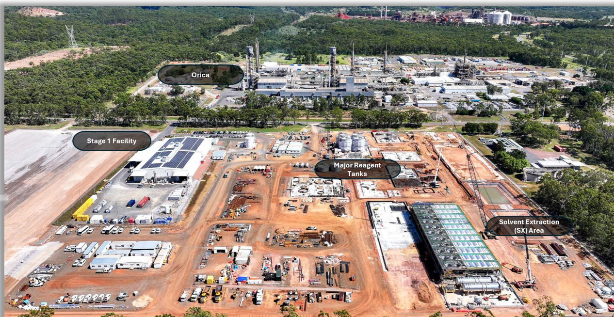
Site-wide image, looking west, showing Stage 2 construction progress
