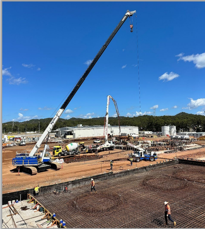
Site civils, looking west (Stage 1 in background)
