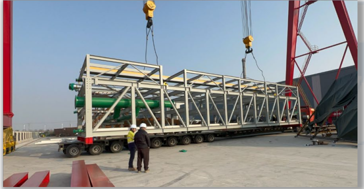
Off-site construction progress showing filtration columns (LHS), motor control centre (MCC) and pipe-rack segment being ship loaded
