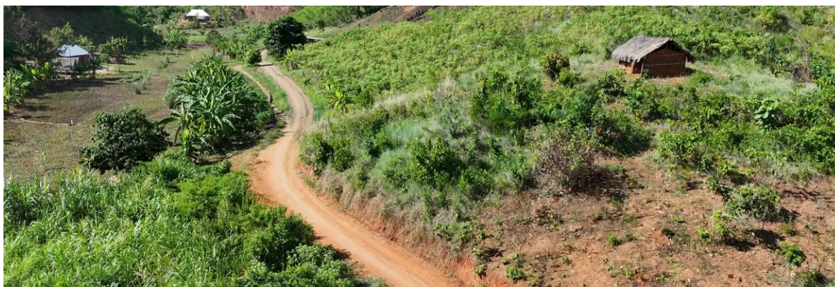
Figure 1: Improvement to farming access track for Mpingu village hamlet.
