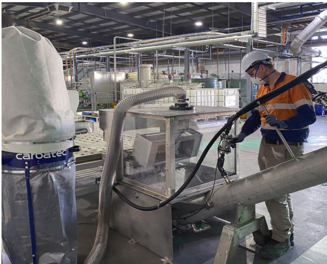
Figure 3. Equipment performance checks at Renascor's PSG demonstration facility
