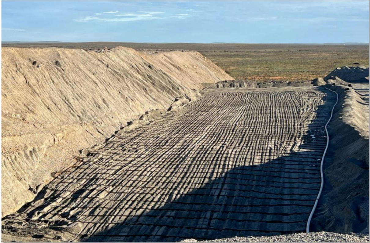
Photo 5: First re-crushed heap leach material now under irrigation
