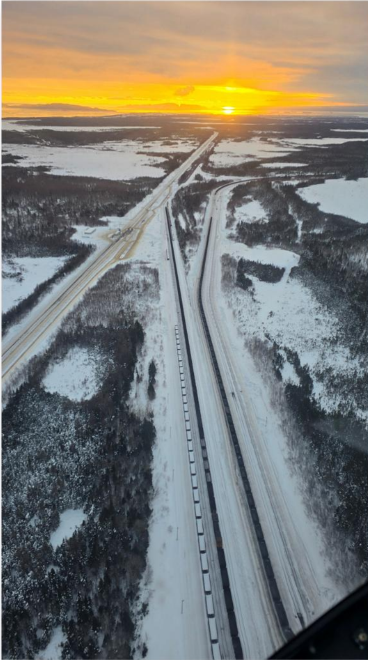
Figure 7. Photo of the existing railroad connecting Sept-Iles to Schefferville
