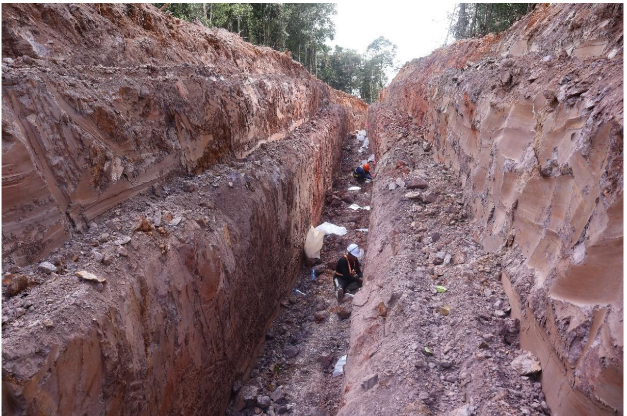
Figure 9: Double benched trenches being employed at SOKO to enter greater sub-soil depths (> 6m) below laterites/duricrust and anomalous levels and well into saprolite/saprock zones which can cut through primary or oxidized mineralisation.
