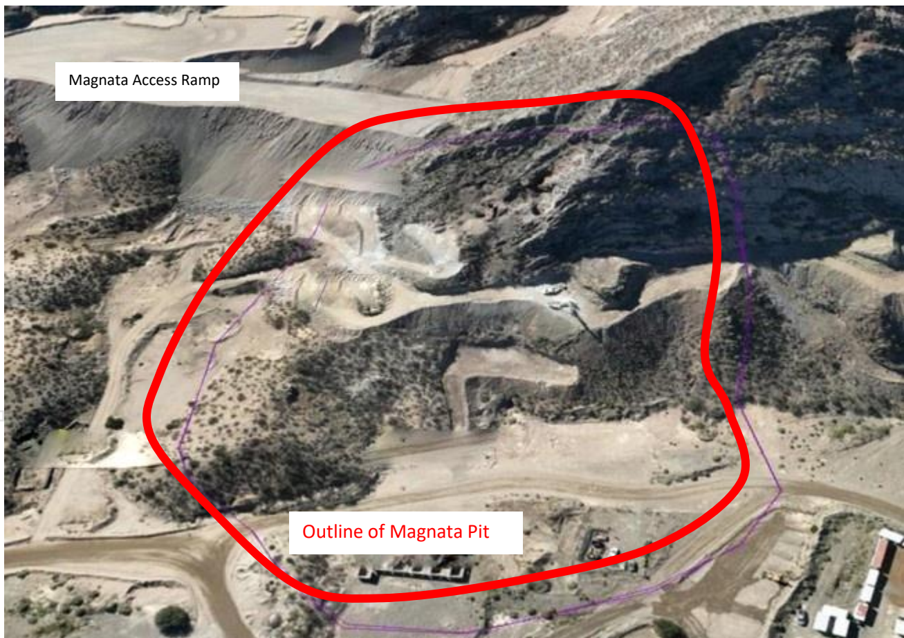
Figure 1 – Showing Magnata Pit and Magnata Access Ramp at 31 March 2026.
