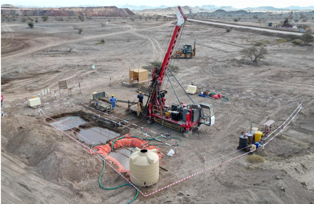
Figure 19: ARL Drilling Site at Al Wash-hi Majaza extension project
