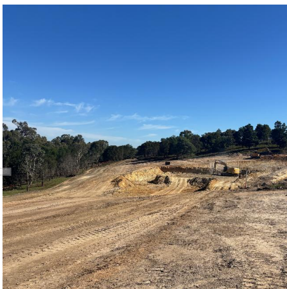
Figure 1. Box cut earthworks, 30 April 2026.
