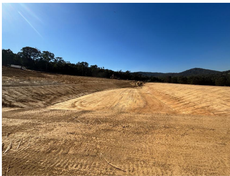
Figure 2. 17 megalitre water dam preparation looking east, note excavator for scale 30 April 2026.
