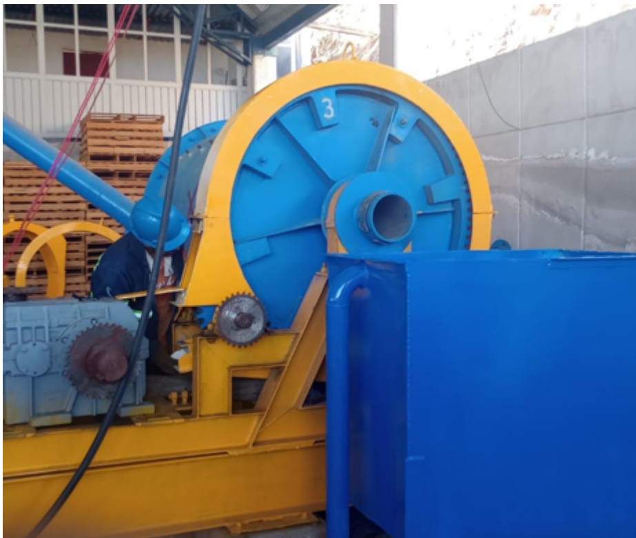
Figure 3: Ball Mill #3 remounted with guards and ore box installed.
