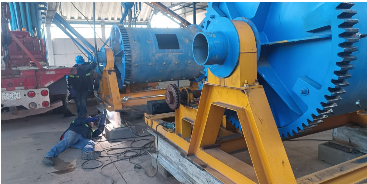
Figure 1 – Completion of Remounting Ball Mill # 1
