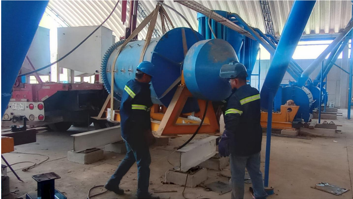
Figure 2 – Mounting of Ball Mill #1.
