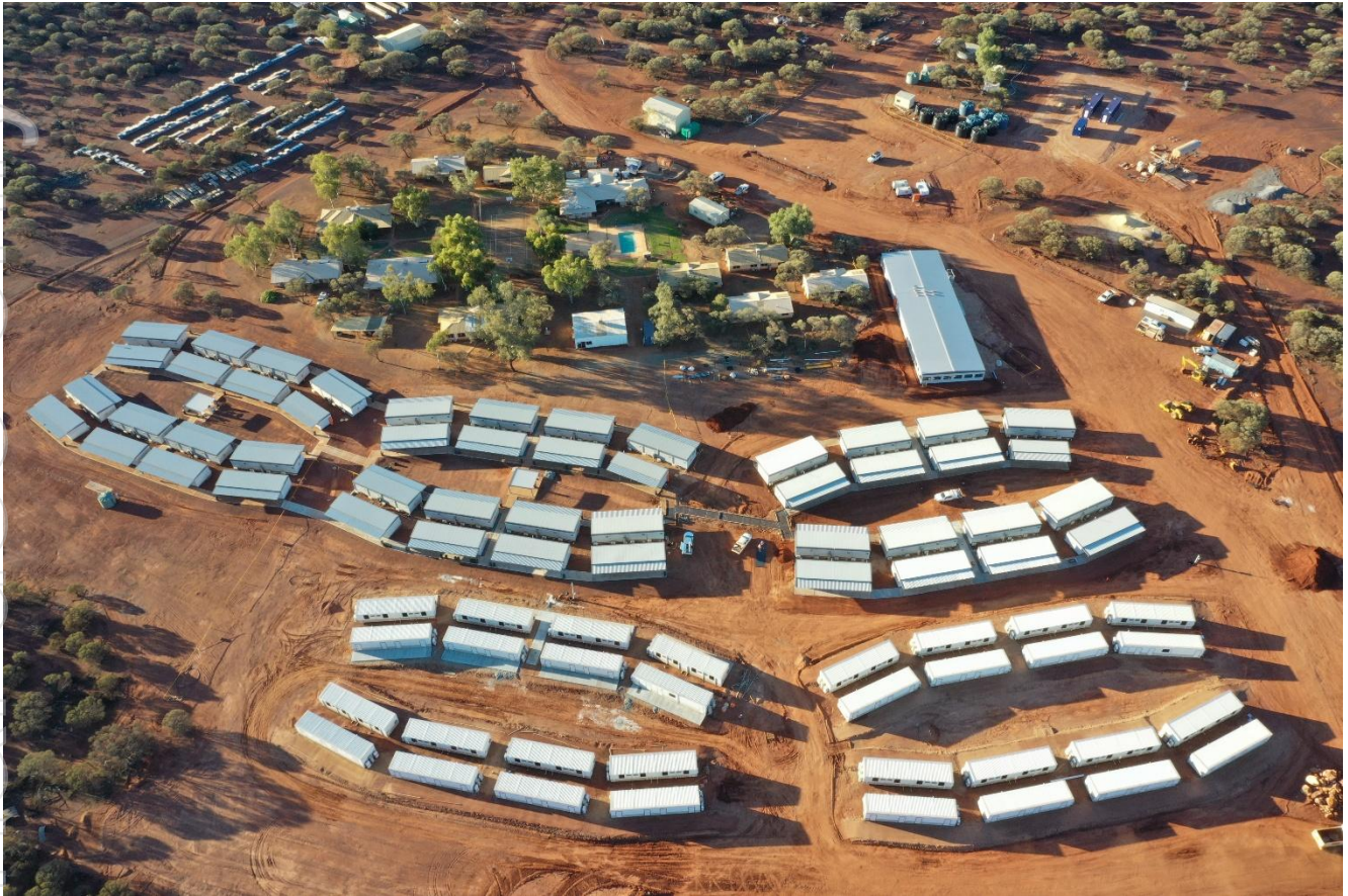
Figure 10 – Camp expansion – all buildings onsite
