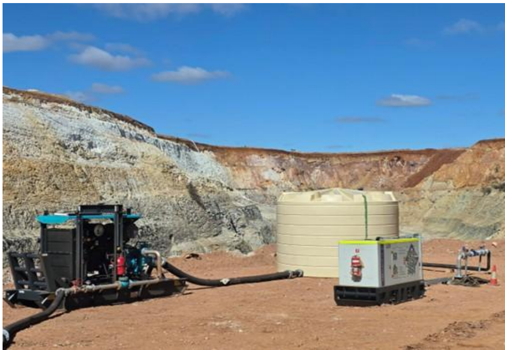
Figure 2 – Youanmi Main initial UG dewatering setup
