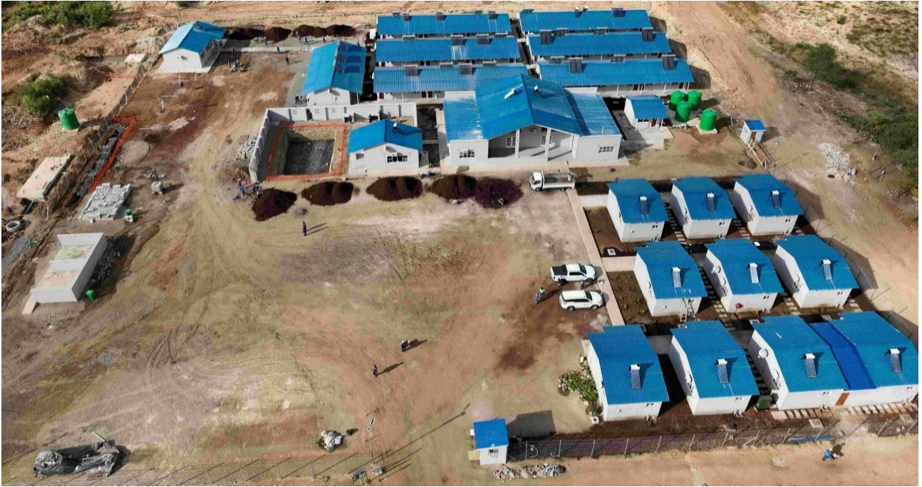
Picture 3. Aerial view of the operational Tipume Camp, which houses 90 personnel
