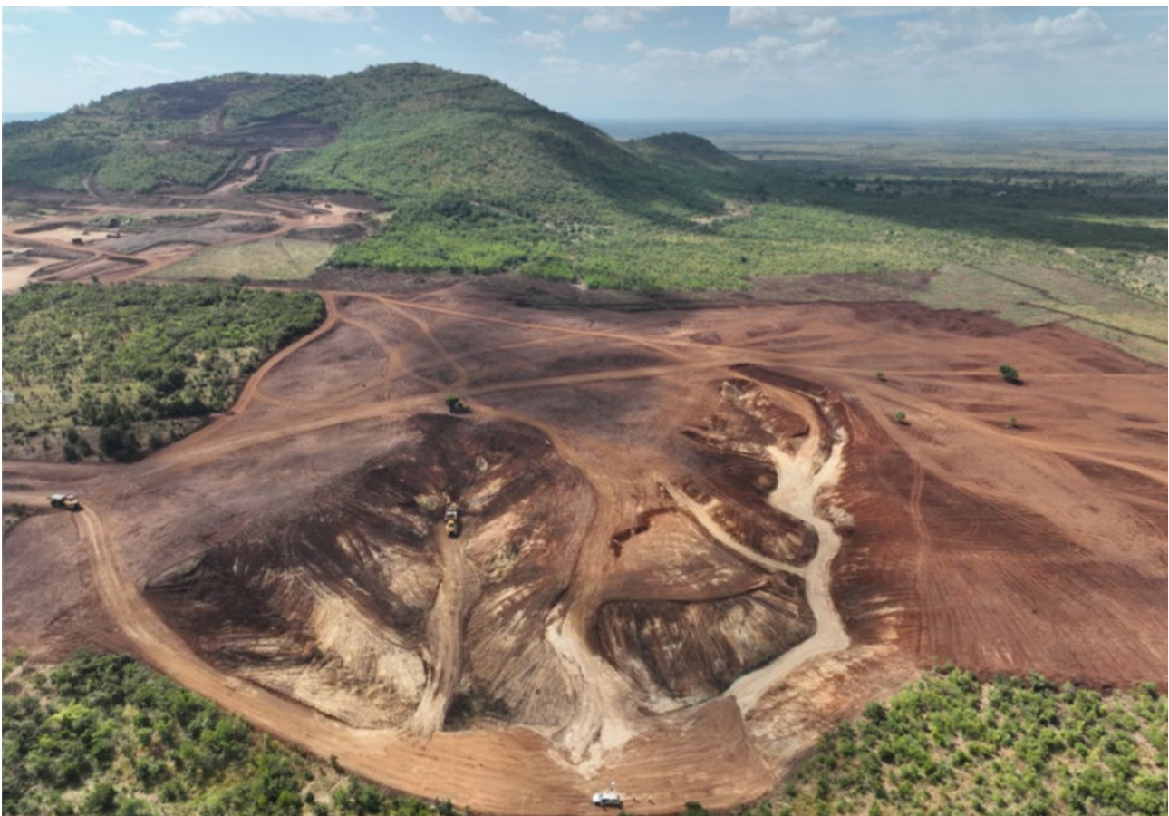
Picture 2. Topsoil Removal at TSF
