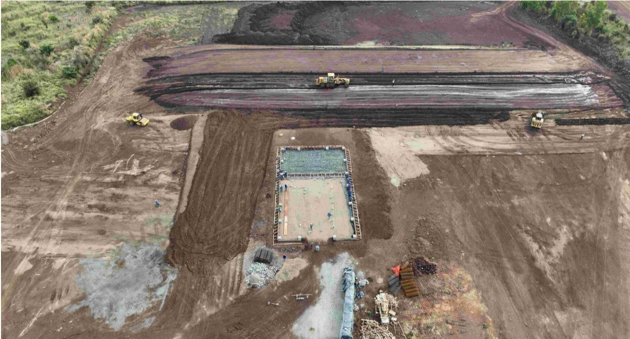
Picture 5. HME Workshop and go line works progressing
