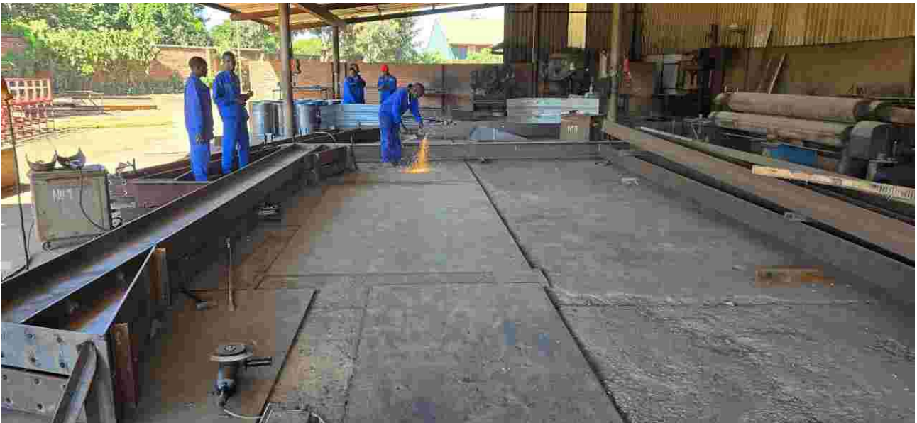
Picture 6. Offsite steel fabrication works
