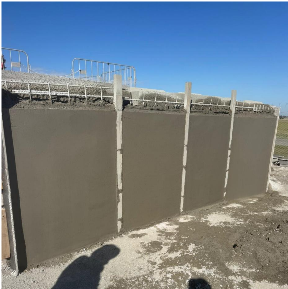
Image 1: Demonstration wall section constructed at Eifers Plant incorporating Eco-Clay
