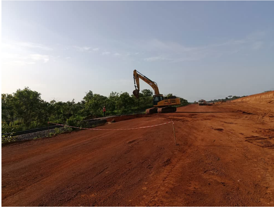
Image 2: Site works at IRF
