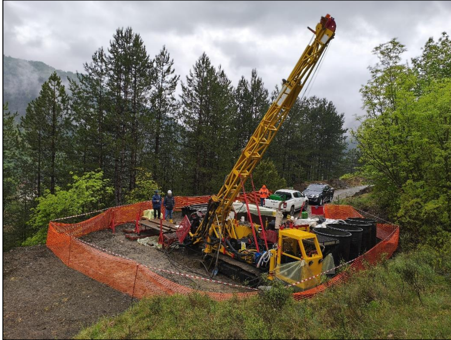
Figure 1. Drilling rig at Ravni Project
