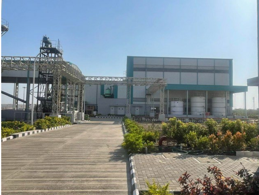
Expandable Graphite JV facility near Pune, India
