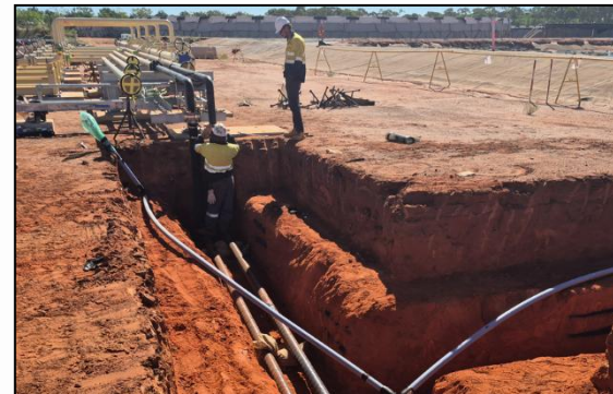
SPCF construction activities (April 2026)
