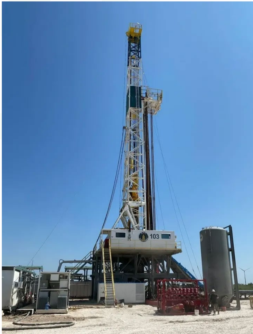
Figure 1: RFC Drilling – Rig 103
