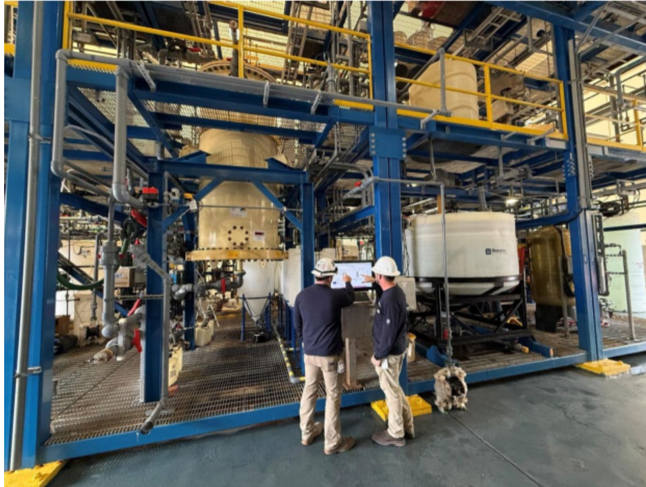
Figure 4: Standard Lithium's single DLE Column in operation in Arkansas (photo from Standard Lithium press release) 1
