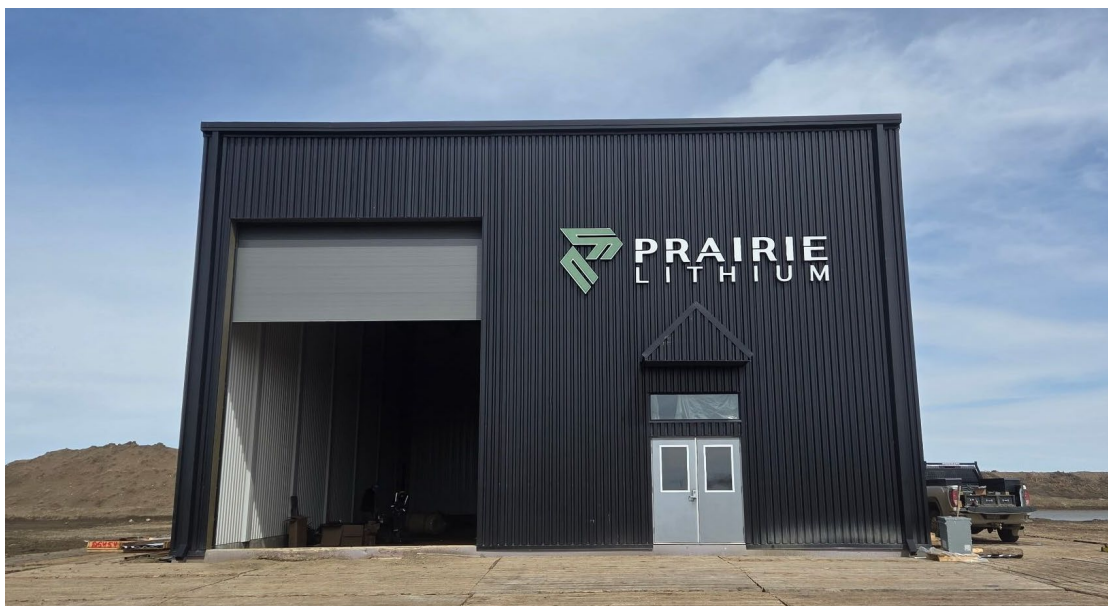
Figure 1: Prairie Lithium's DLE Production Facility in Saskatchewan, Canada
